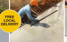
C15/GEN2 CONCRETE Normally used for pavement kerbs and floor blinding.
