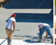
C20/GEN3 CONCRETE Frequently used for paving and slab foundations.
