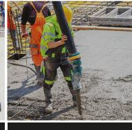
C40 CONCRETE Usually used for commercial slabs and structural piling.
