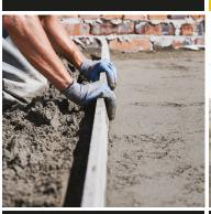
**CONCRETE FLOOR SCREED** Commonly used for screeding an internal or external floors.
